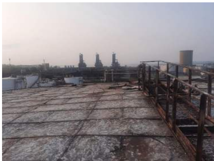
Fig. 5.3 Corroded sheet protection (source author))
