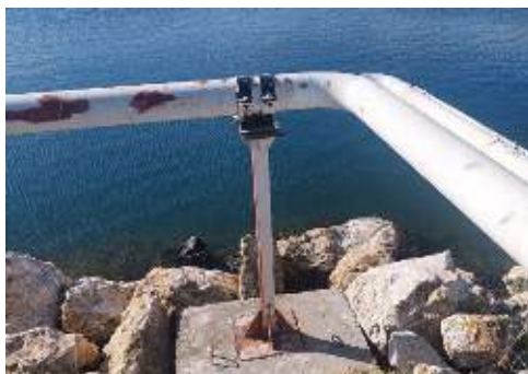
Fig 5.6, 5.7 poor technical condition of pipelines (source author)
