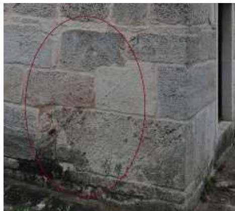
Fig.3.3. The cracking and disintegration of masonry stones – Esmahan Sultan mosque (author's photo)
