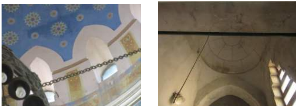
Fig.3.5. Carol I Mosque – degraded areas on the dome (author’s photo)
