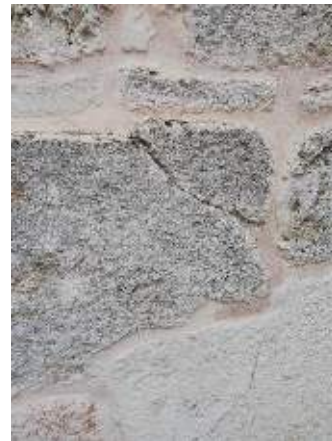
Fig.3.3. The cracking and disintegration of masonry stones – Esmahan Sultan mosque (author's photo)
