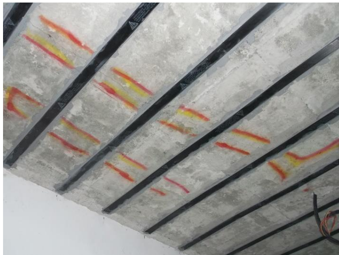
Figure. 4.5 Consolidation of the floor with composite strips (personal archive photo - Maritime University of Constanța - building Nautical Base)
