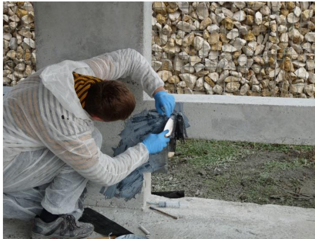
Figure. 4.10 Consolidation of zone 2 with composite anchors
