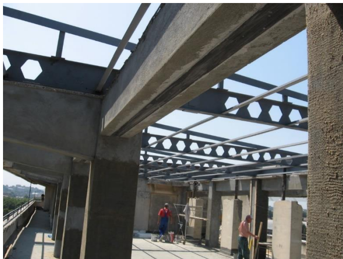
Figure. 4.4 Final repairs with composite systems to damaged elements (personal archive photo - Maritime University of Constanța)
