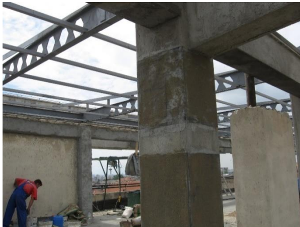
Figure. 4.6 Final repairs with composite systems at the columns (personal archive photo - Maritime University of Constanța)
