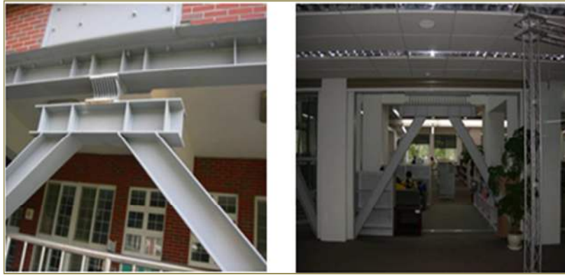
Figure 3.1.1 „Building equipped with ADAS type shock absorber” (Cheng, 2008)
