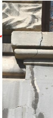
Figure 3.19 – Museum of National History and Archeology – Constanta - detail cracked front side – photo 2008 –
