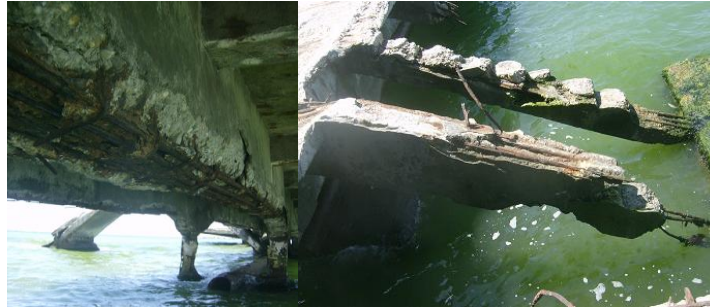
Figure 3.13, 3.14- Degraded concrete elements at Casino Mamaia walkway (author photo)
