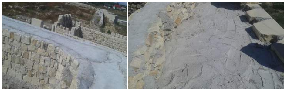
Figure 5.35, 5.36- Rehabilitation of Capidava Citadel walls using conventional concrete (author photo)
