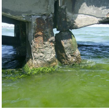
Figure 3.16- Concrete elements subjected to the action of vegetation
