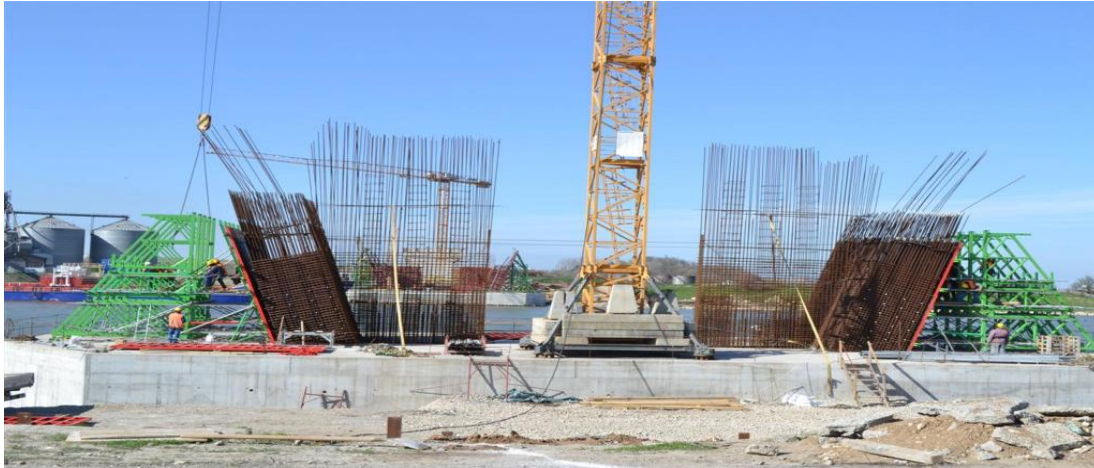
Figure 4.39- Elements before casting, in "Bridge over the Danube-Black Sea Channel, km 0 + 540" project (author photo)
