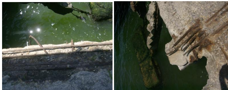
Figure 5.20, 5.21- Damage of concrete elements on Casino Mamaia walkway (author photo)
