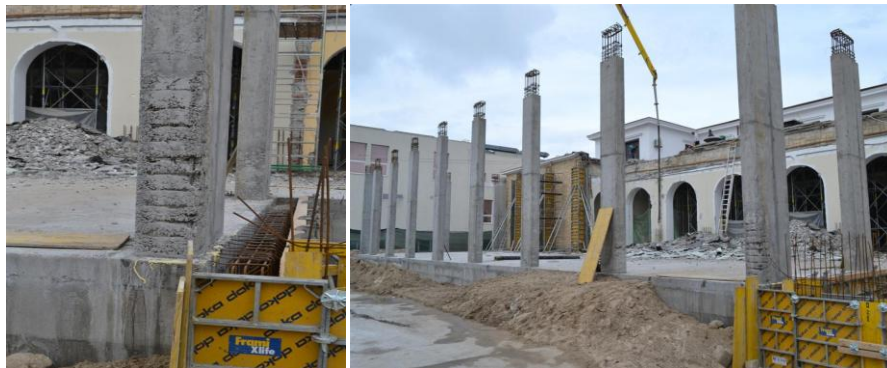
Figure 4.33, 4.34- Construction elements poorly compacted due to large height of elements (photo author)
