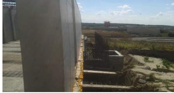
Figure 5.37-Construction element of self compacted concrete at Capidava Citadel (author photo)
