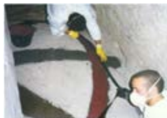
Fig. 3.54 - Solutions to restore masonry arches with composite materials - (photo João Appleton, João Ferreira)
