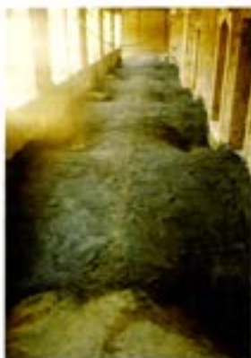
Fig. 4.5 - Jacketing of masonry vaults polymer mesh - (photo João Appleton)
