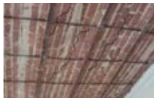
Fig. 3.36 - Cracks in brick masonry vaults - (photo author)
