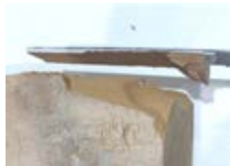
Fig. 4.67 - Posting CFRP strips of bricks - (photo author)
