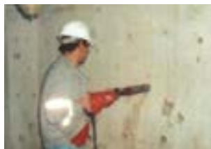
Fig. 3.9 – Carotaj technique – (photo Vítor Cóias)
