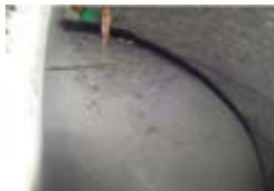
Fig. 3.50 - Crack clogging with resins or foams - (photo author)
