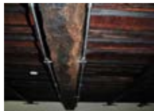
Fig. 3.28 - Strengthening wooden floor with platbens and metallic ties - (photo João Appleton)
