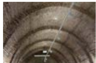
Fig. 2.26 – Cylindrical vault with masonry ribs - (author photo)
