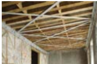
Fig. 3.24 - Strengthening connections between floor wooden beams and walls - (photo João Appleton)
