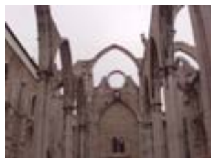
Fig. 3.43 – Vaults collapsed due to seismic action - Carmo Church / Lisbon - (photo author)
