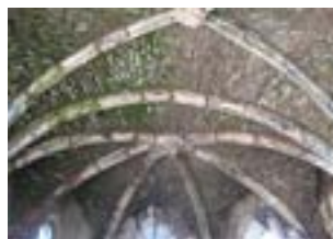
Fig. 2.8 – Brick floor – Vela vault – (author photo)
