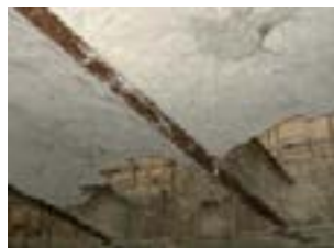
Fig. 3.36 - Cracks in brick masonry vaults - (photo author)
